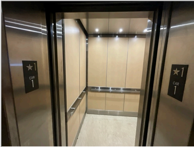
LOBBY LOOKING AT CABS
