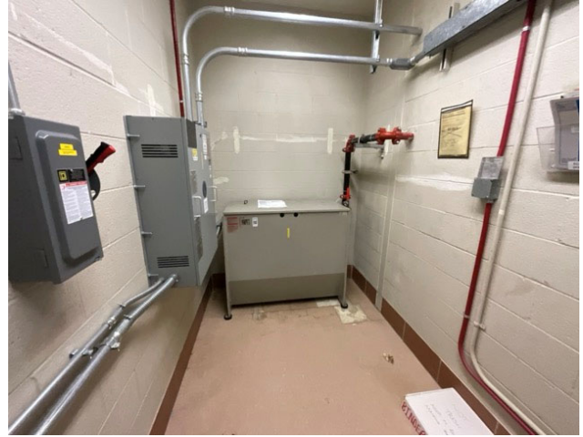
20 - ELEVATOR MACHINE ROOM
