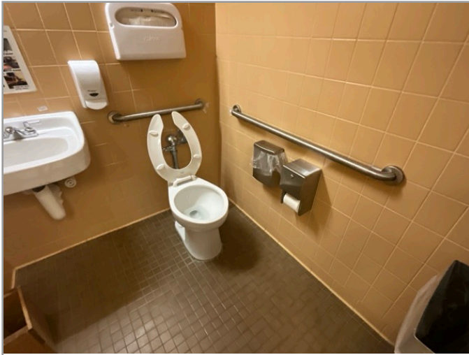
TOILET STALL OVERVIEW
